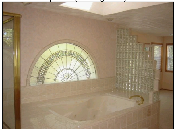
Figure 6 – Shower and Tub Enclosures In this example, the shower enclosure at the left contained tempered safety glass, and the glass blocks at the end of the tub are exempt. The leaded glass next to the tub is not allowed; any windows in that area must be safety glass.
